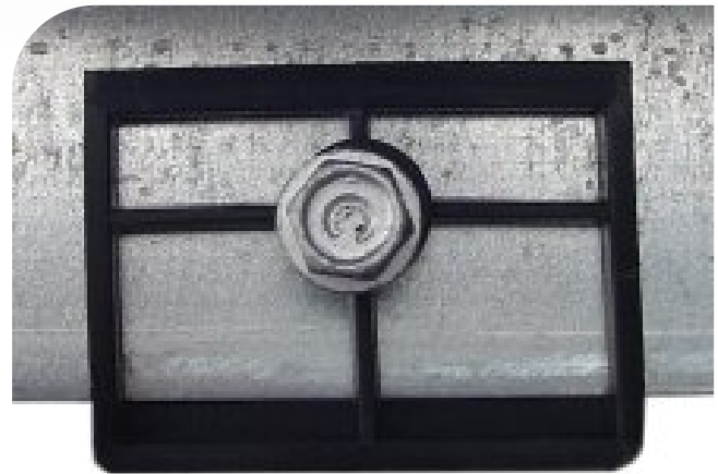
Fig 1: Under driven – cross hairs not deformed
