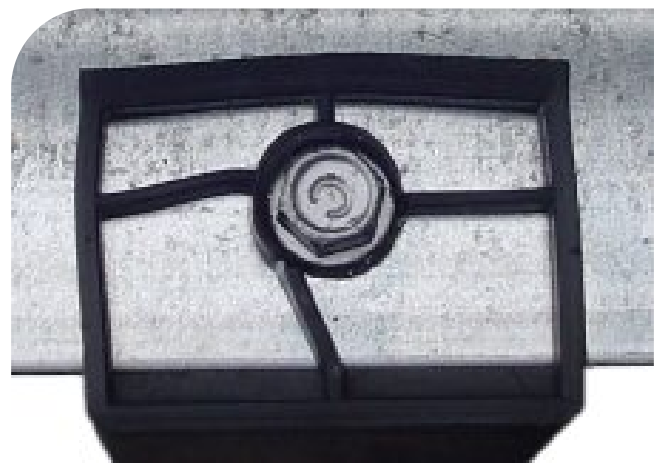
Fig 3: Correctly driven – cross hairs deformed but not snapped
