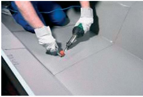
Sealing Cascade gutter sole joint
