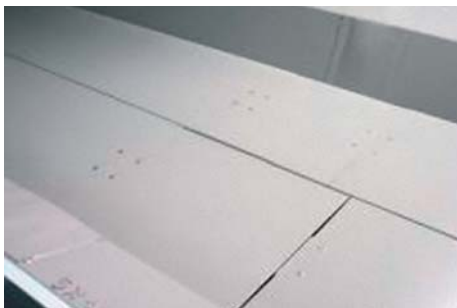
Second Transition piece installed
