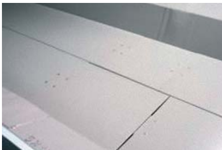
Second Transition piece installed
