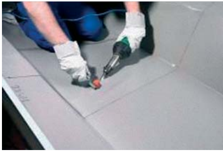
Sealing Cascade gutter sole joint
