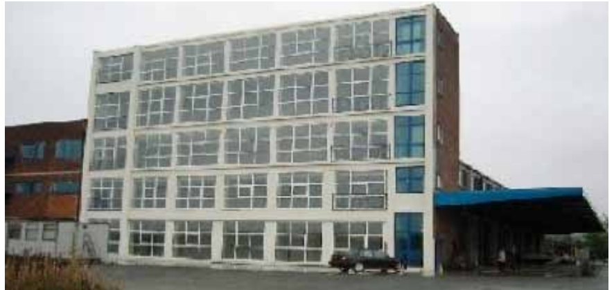
Figure 24. Building before pre-finished steel rainscreen over cladding system
