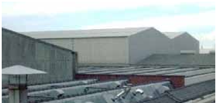
Figure 15. Before refurbishment of the building
