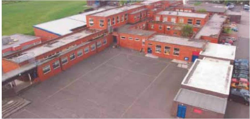
Figure 21. School before refurbishment of the flat roof
