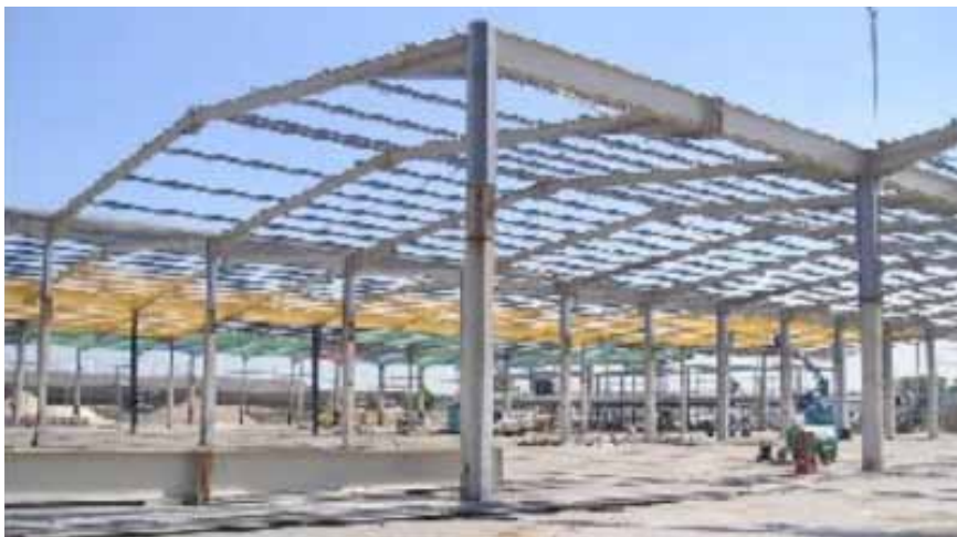
Figure 7. Refurbished portal frame ready for re-sheeting
