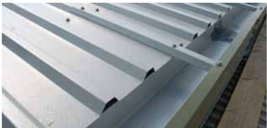
Figure 18. Roof after refurbishment showing pre-finished steel composite panel roof cladding
