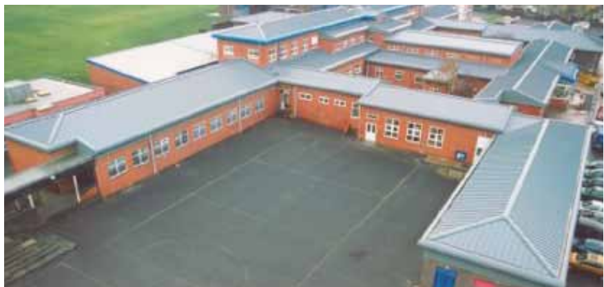
Figure 22. School after pre-finished steel flat to pitch roof system refurbishment
