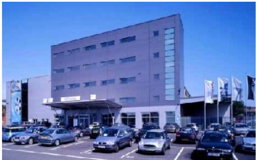
Figure 25. Building after pre-finished steel rainscreen over cladding system
