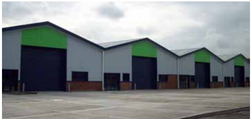
Figure 20. Industrial buildings after refurbishment
