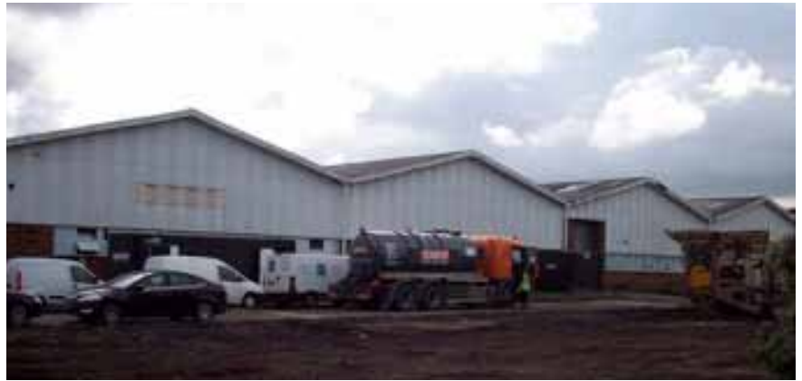
Figure 19. Industrial buildings before strip and re-sheet
